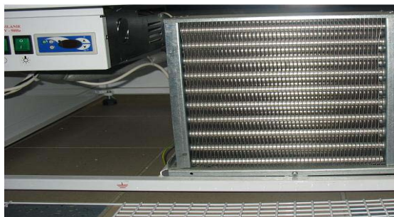
Fig.10 Cleaning the condenser
